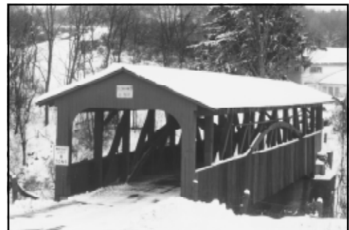
Covered Bridge in Luthers Mills, Bradford County, PA
