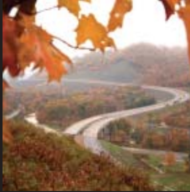
The I-99 corridor nears completion in Tioga County
