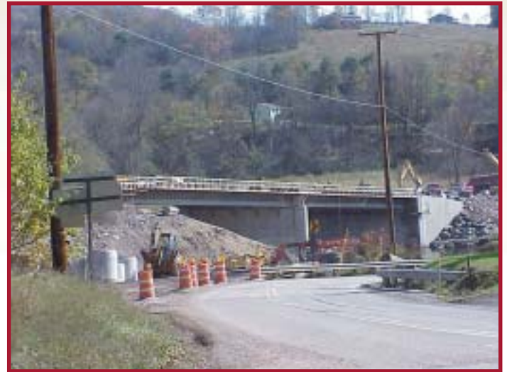
Bridge replacement of SR 3023 in Rush Township, Susquehanna County.
